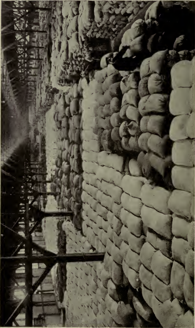
View of a Grain Storage at Hamburg.
